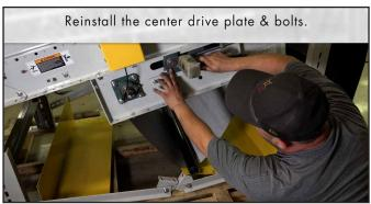
Reinstall the center drive plate & balls.
